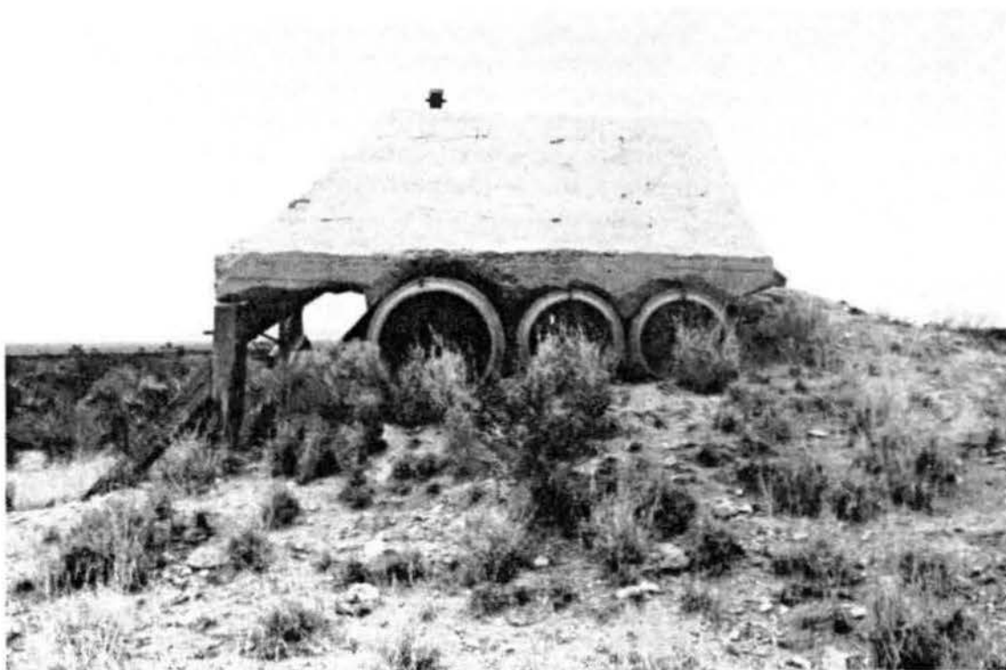
Remains of North 800 bunker (HSR photograph file).
