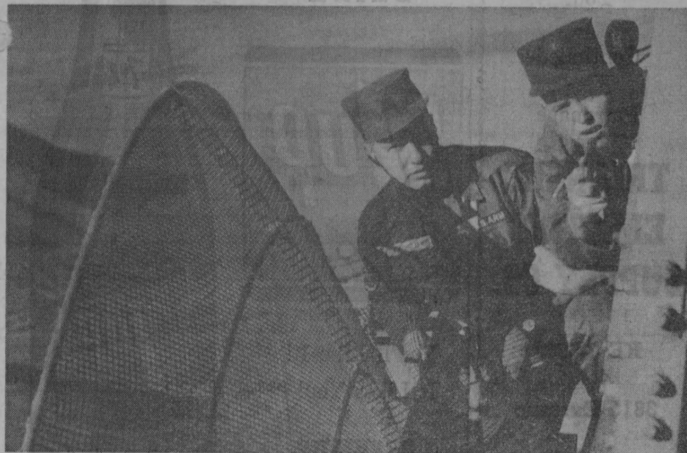
VIEW FROM THE TOP —Two miles high at North Oscura Peak station, soldiers of the Signal Missile Support Agency work on a microwave antenna tower used in the data transmission system on the missile range at White Sands. (U.S. Army photo)
