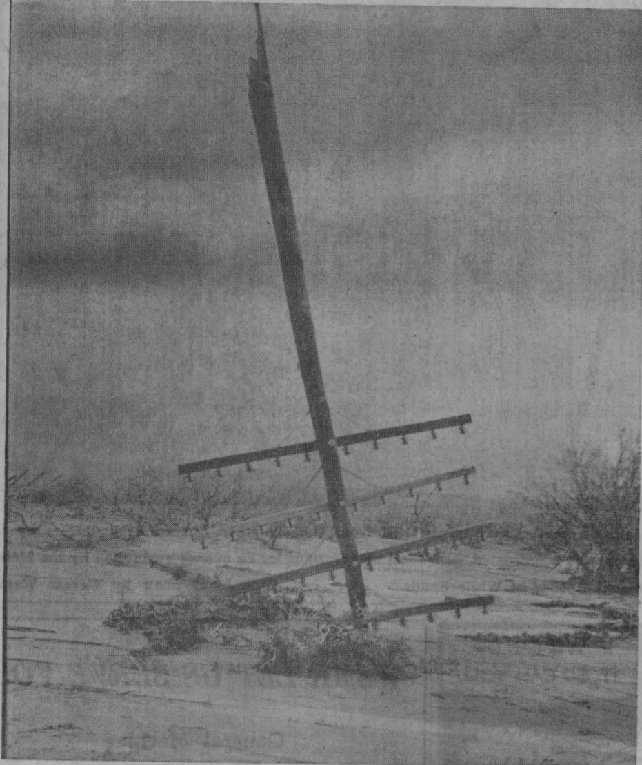
HIGH WINDS BLOW —Here's what sometimes happens to pole lines at White Sands Missile Range when the big winds come. Signal Missile Support Agency soldiers rush into action to repair the damage in hours. (U.S. Army Photo)
